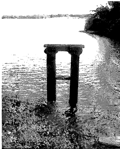
FIGURE 4.13: Sluice operating platform located in water spread area.
