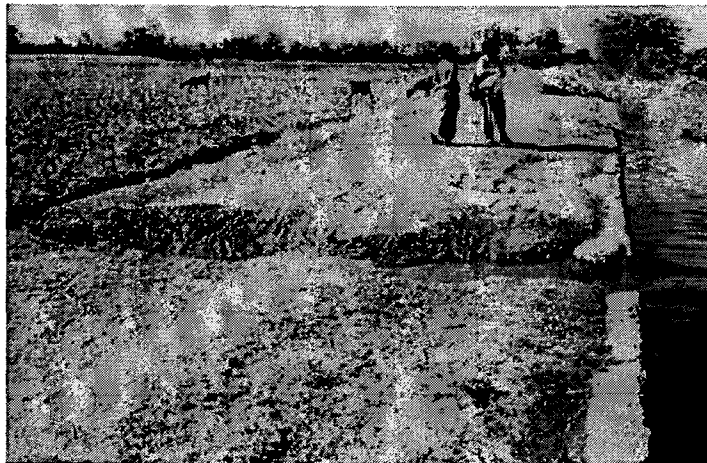
FIGURE 8.2: An open channel taking off from the main canal.
